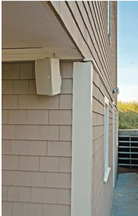
Figure 2. Placing speakers on the house provides sound to the deck, to the yard, and perhaps to the neighbor's yard. Speakers facing inward from the deck's perimeter take a little more wire, but the sound stays on the deck.
