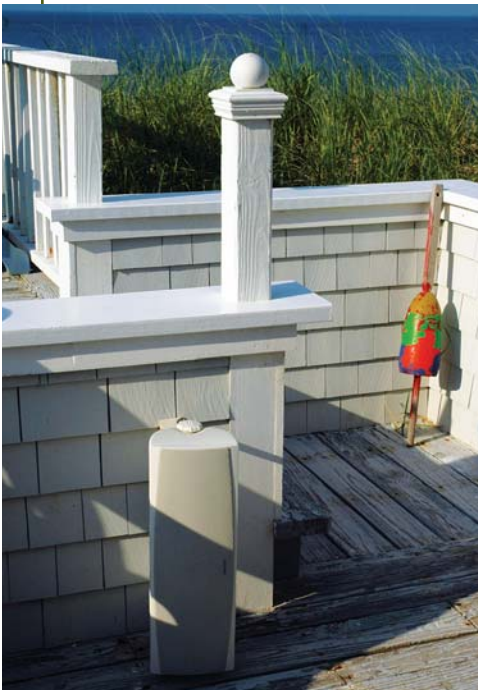
Figure 5. Walled-in decks provide the best opportunity for hiding speaker wires. Otherwise, the wires generally run inside newel post sleeves.
